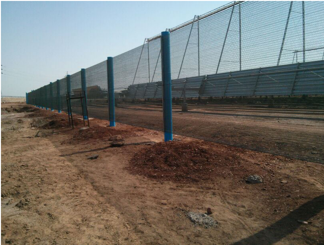
Solar Array Wind and Dust Protection
