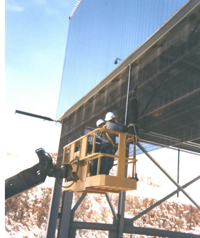
Crusher Building and Transfer Tower Siding
