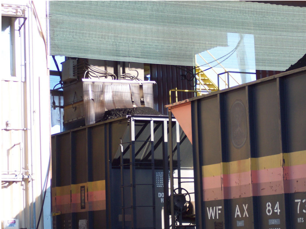
Rail Load out Building
